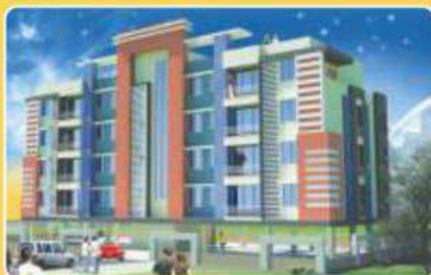
Katayni Enclave Near RPS School, Bailey Road, Patna
