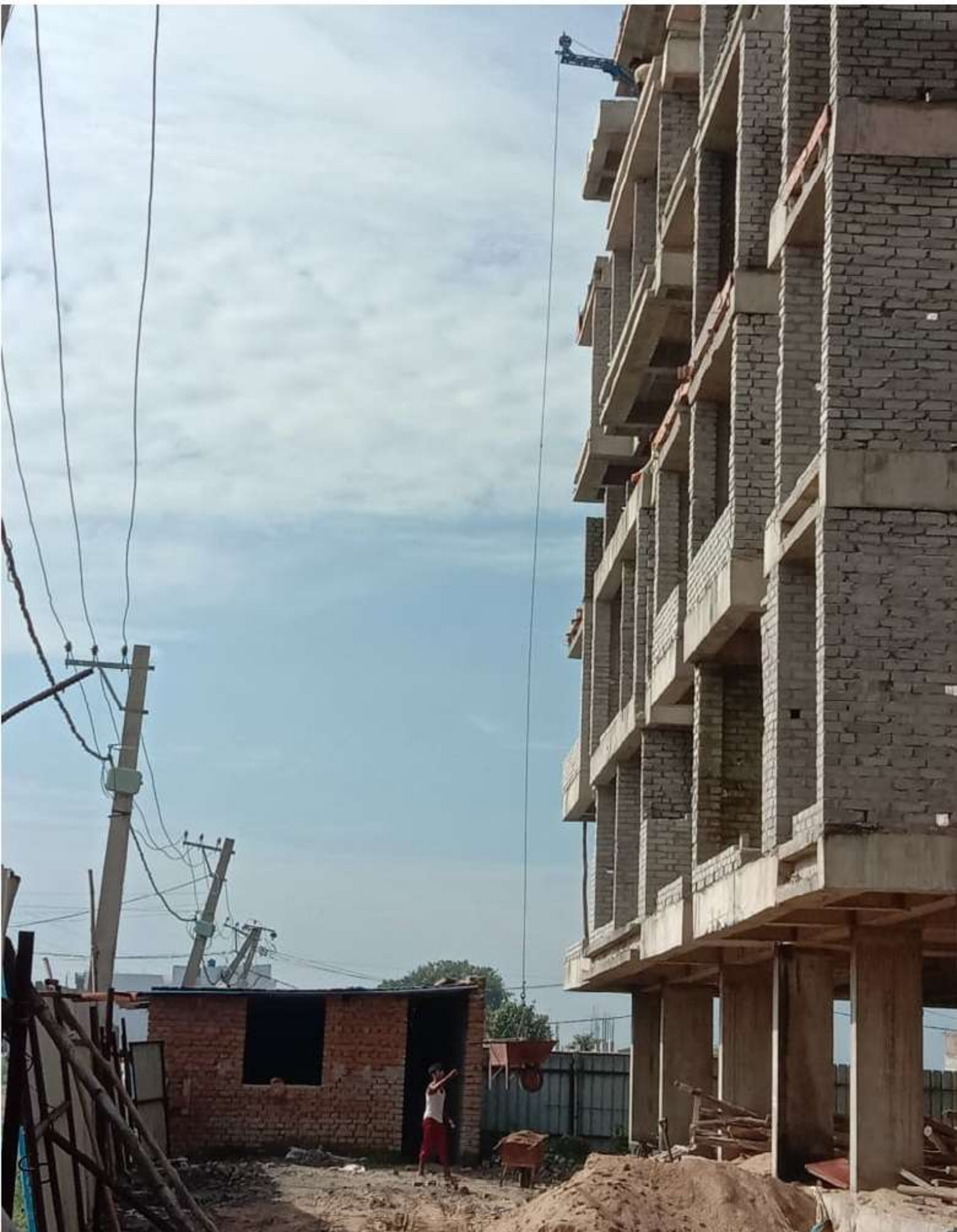
BLOCK -A 1ST FLOOR, 2ND FLOOR, 4TH FLOOR BRICK WORK COMPLETED
