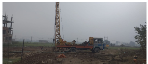
TOWER 2 PILE CASTING IN PROGRESS
