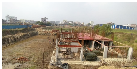
RAFT BOTTOM MAT REINFORCEMENT WORKS
