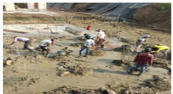
PILE BREAKING , SOLING AND PCC
