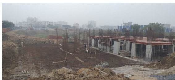
COLUMN STEEL WORKS IN RAFT AREA
