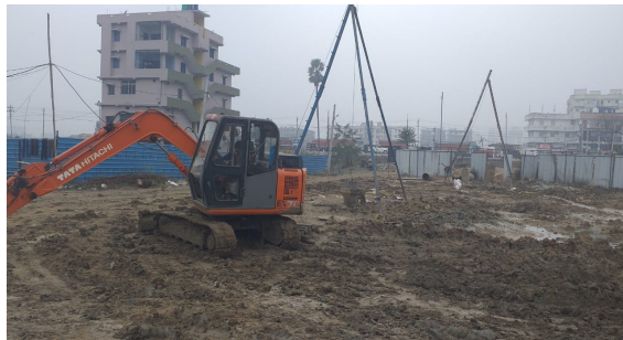
MALL AREA PILE CASTING IN PROGRESS
