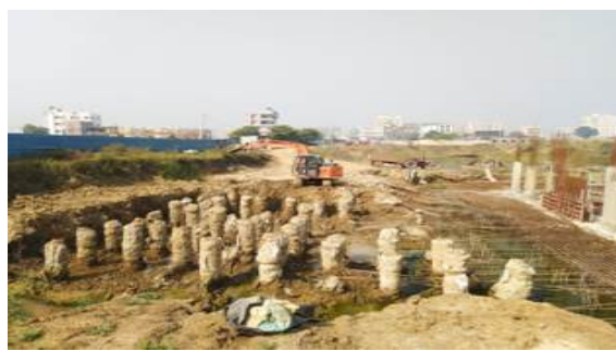
PILE AREA EXCAVATION WORKS
