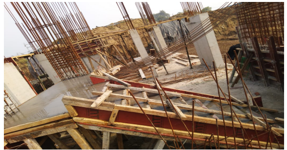
CASTING OF BASEMENT SLAB
