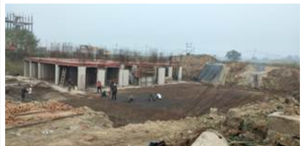
RAFT AREA REINFORCEMENT TOP MAT WORKS
