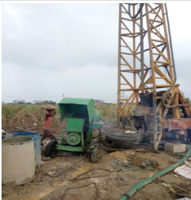
Pile Casting work
