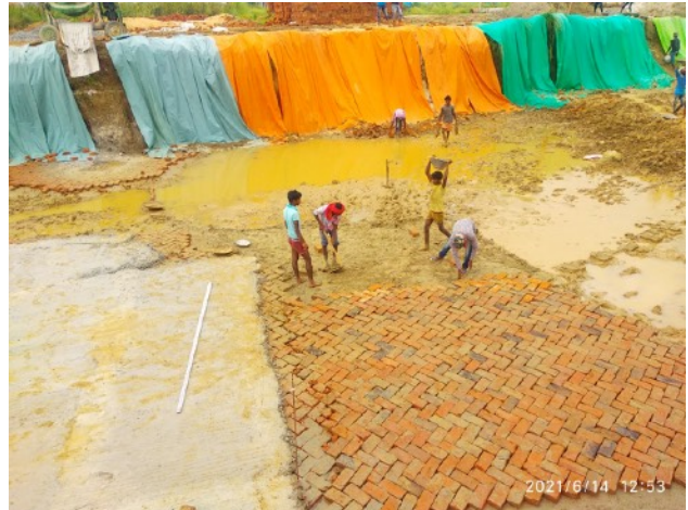
Bricks soling work
