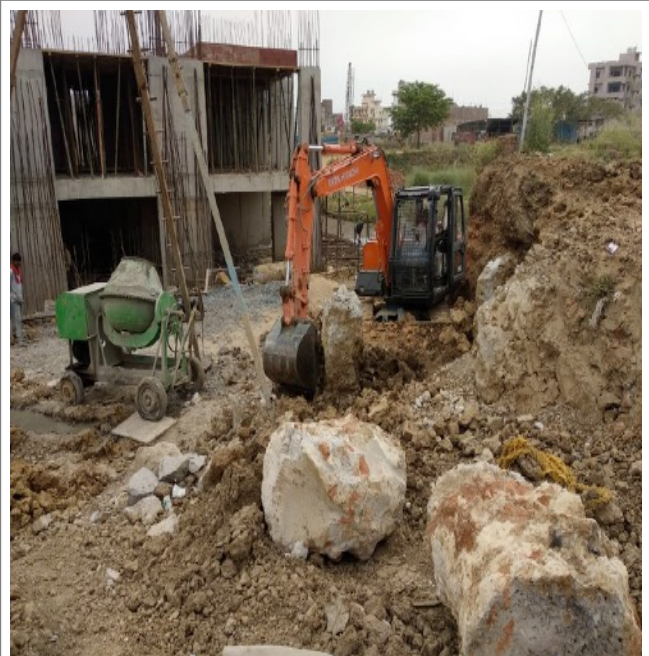
Soil excavation work
