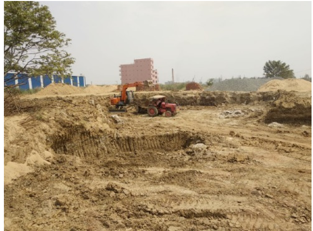
Soil Excavation work
