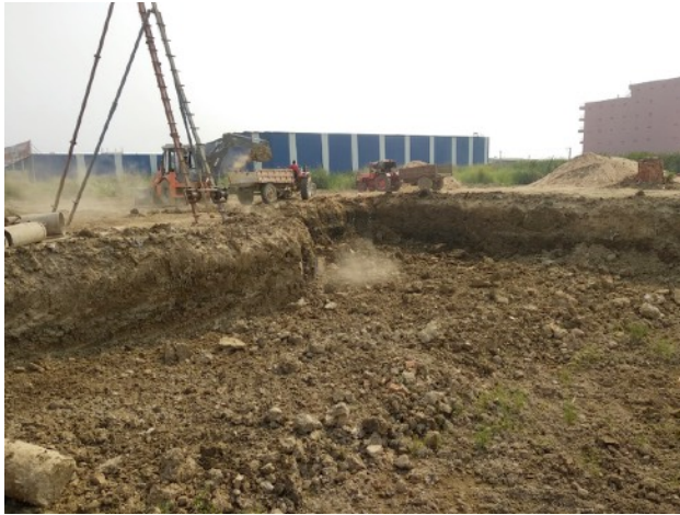
Soil Excavation work
