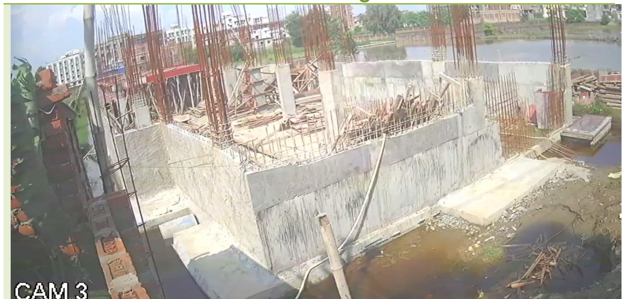
Construction Status Images of Block -B
