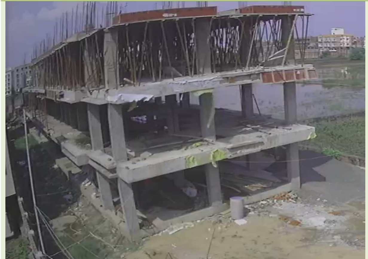
Construction Status Images of Block -A
