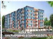
Completed RAJDEV ENCLAVE A | B
