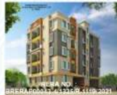
Completed RAJDEV ENCLAVE C
