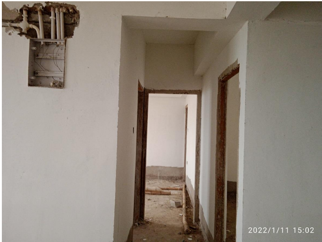
Internal Putty Work.
