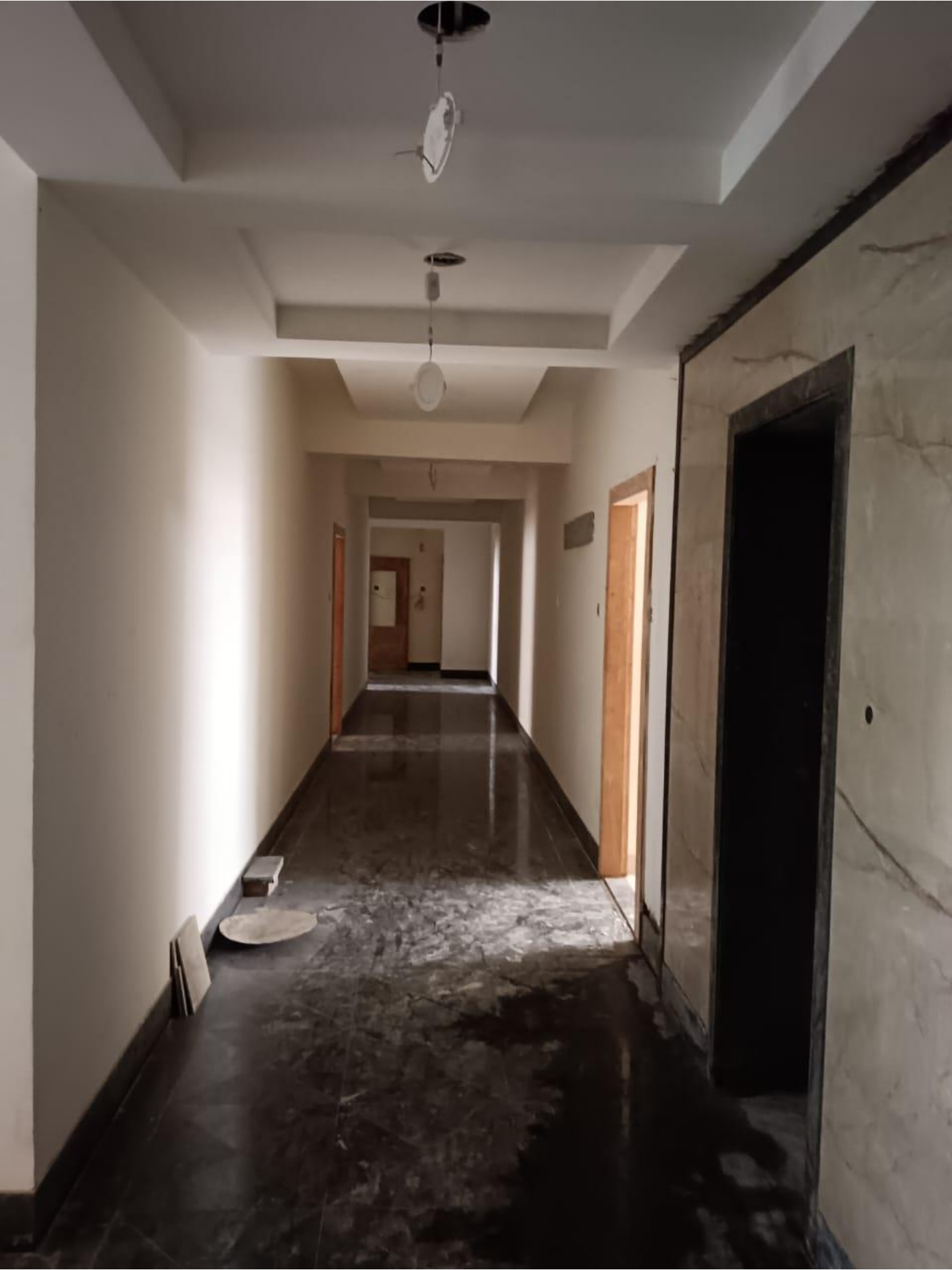
1 ST FL LOBBY
