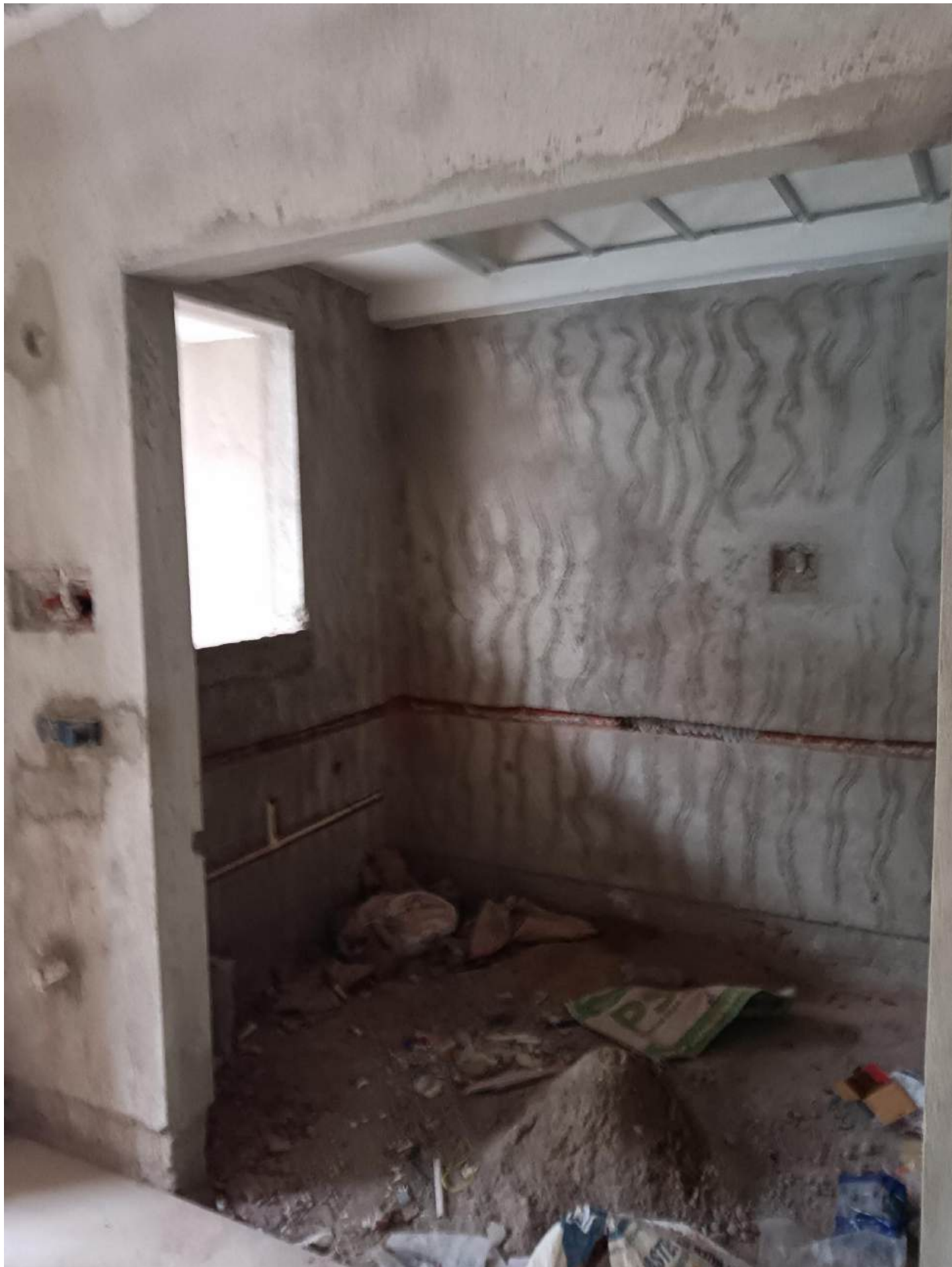
1 ST FL. KITCHEN
