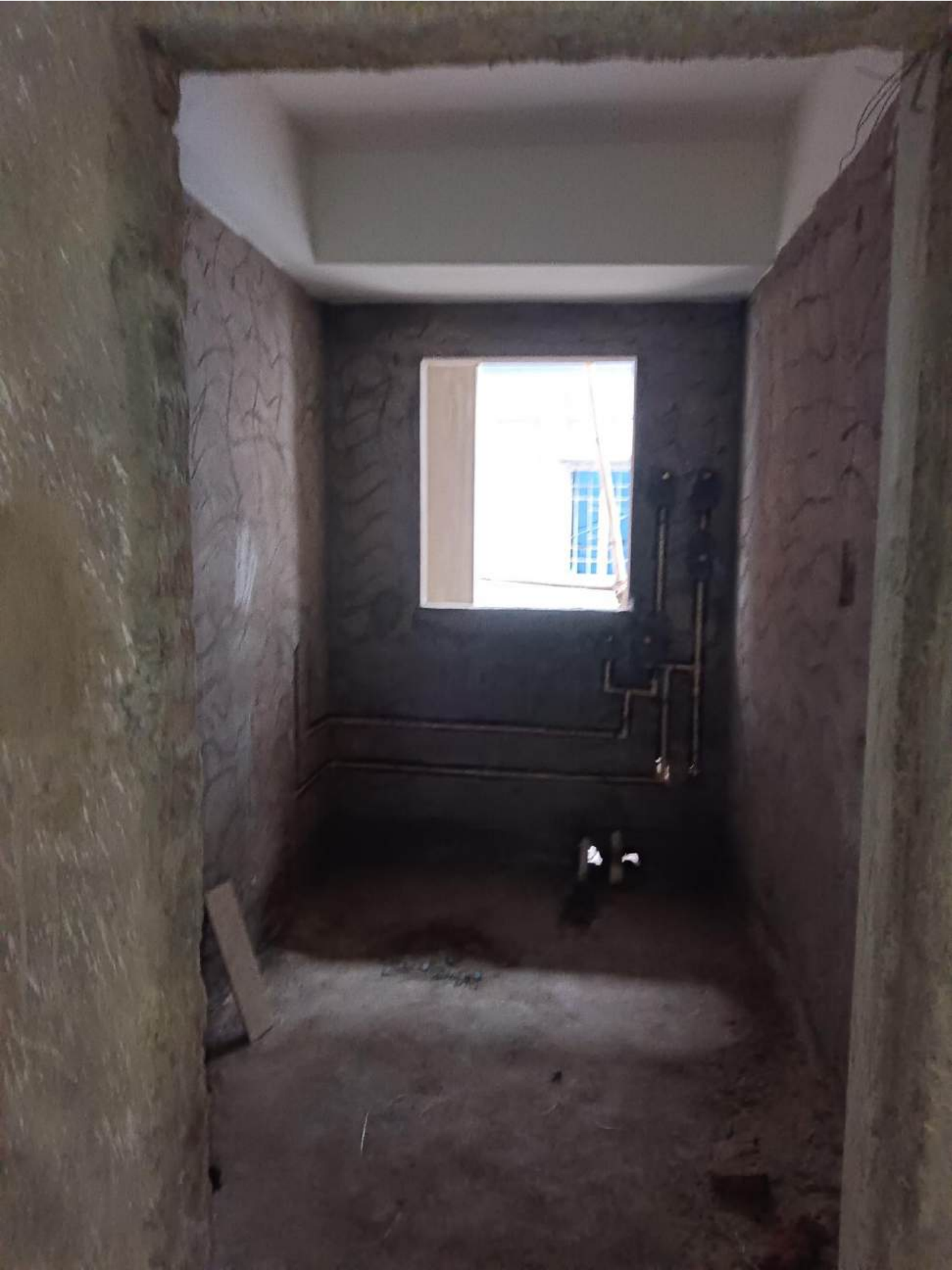
1 ST FLOOR BATHROOM
