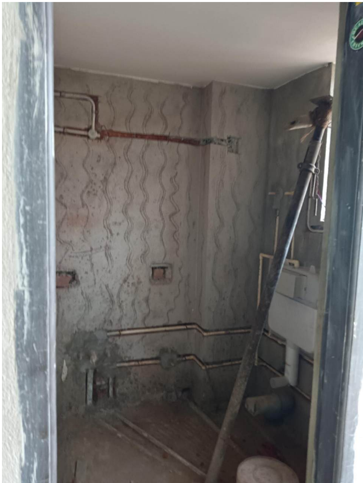
2 ND FL BATHROOM
