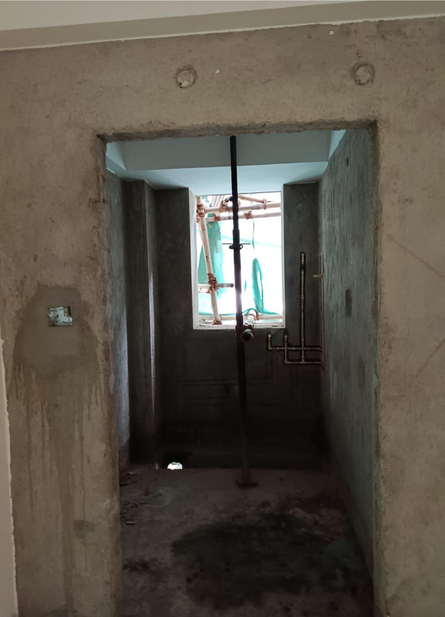
1 ST FL. KITCHEN
