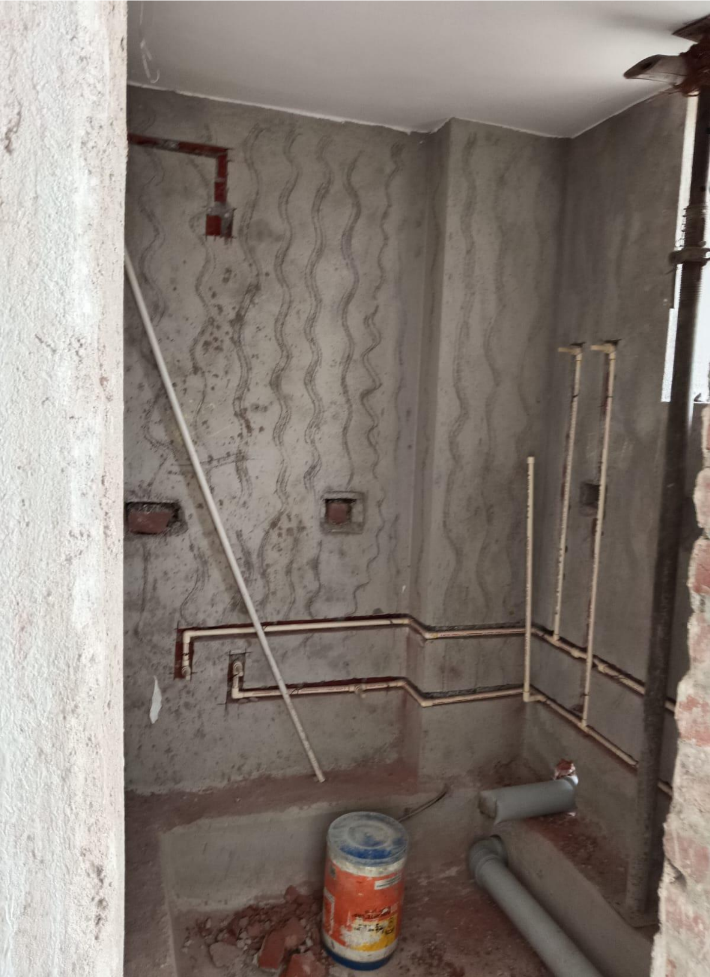
2 ND FL BATHROOM
