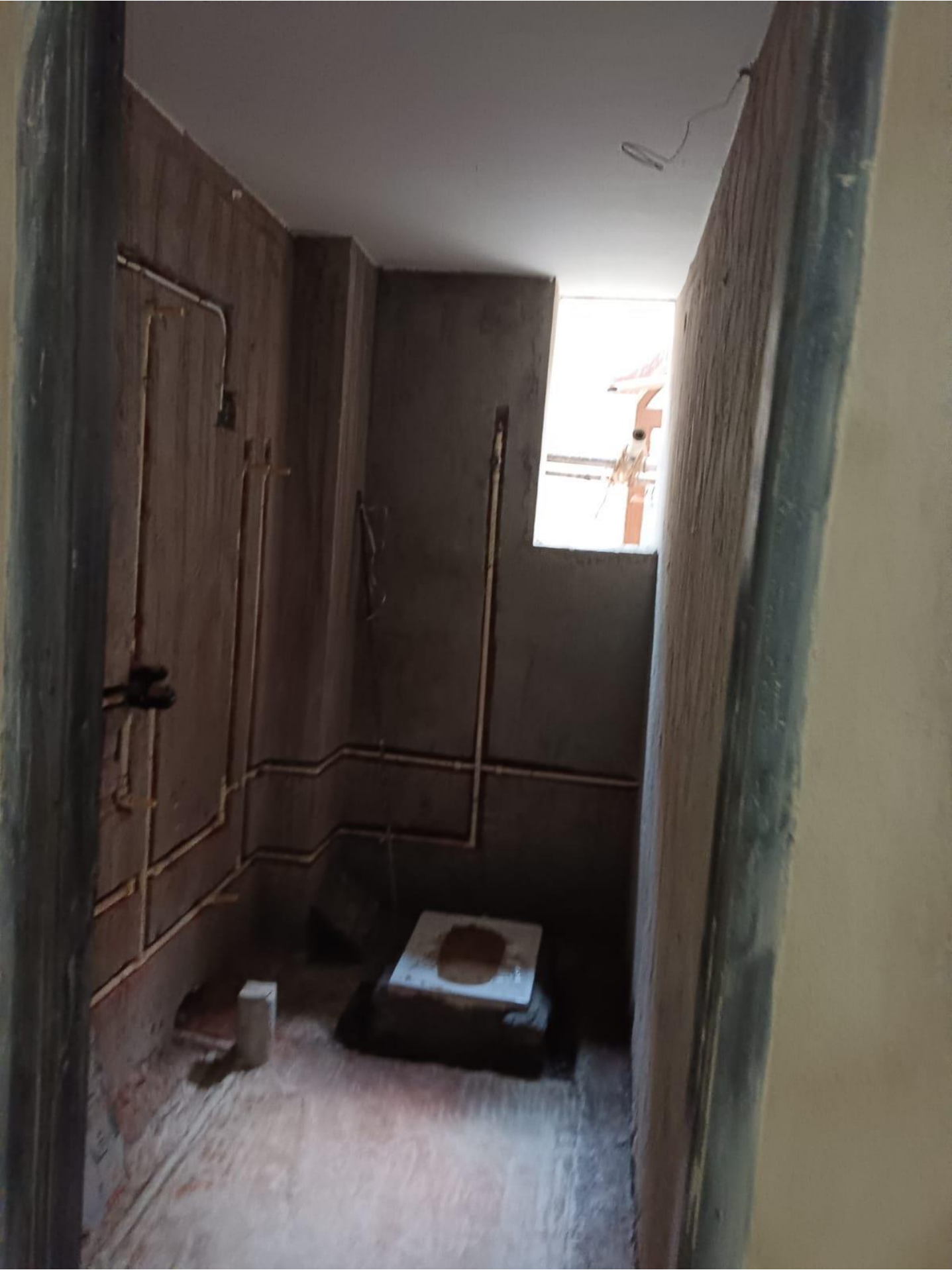
1 ST FLOOR BATHROOM
