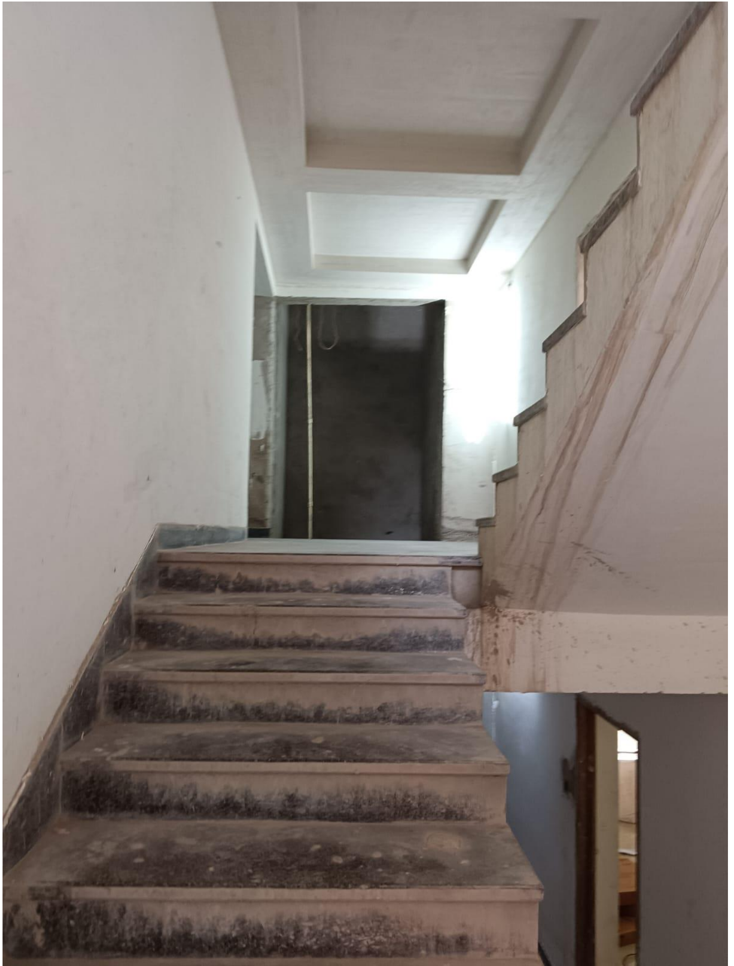
2 ND FL STAIR
