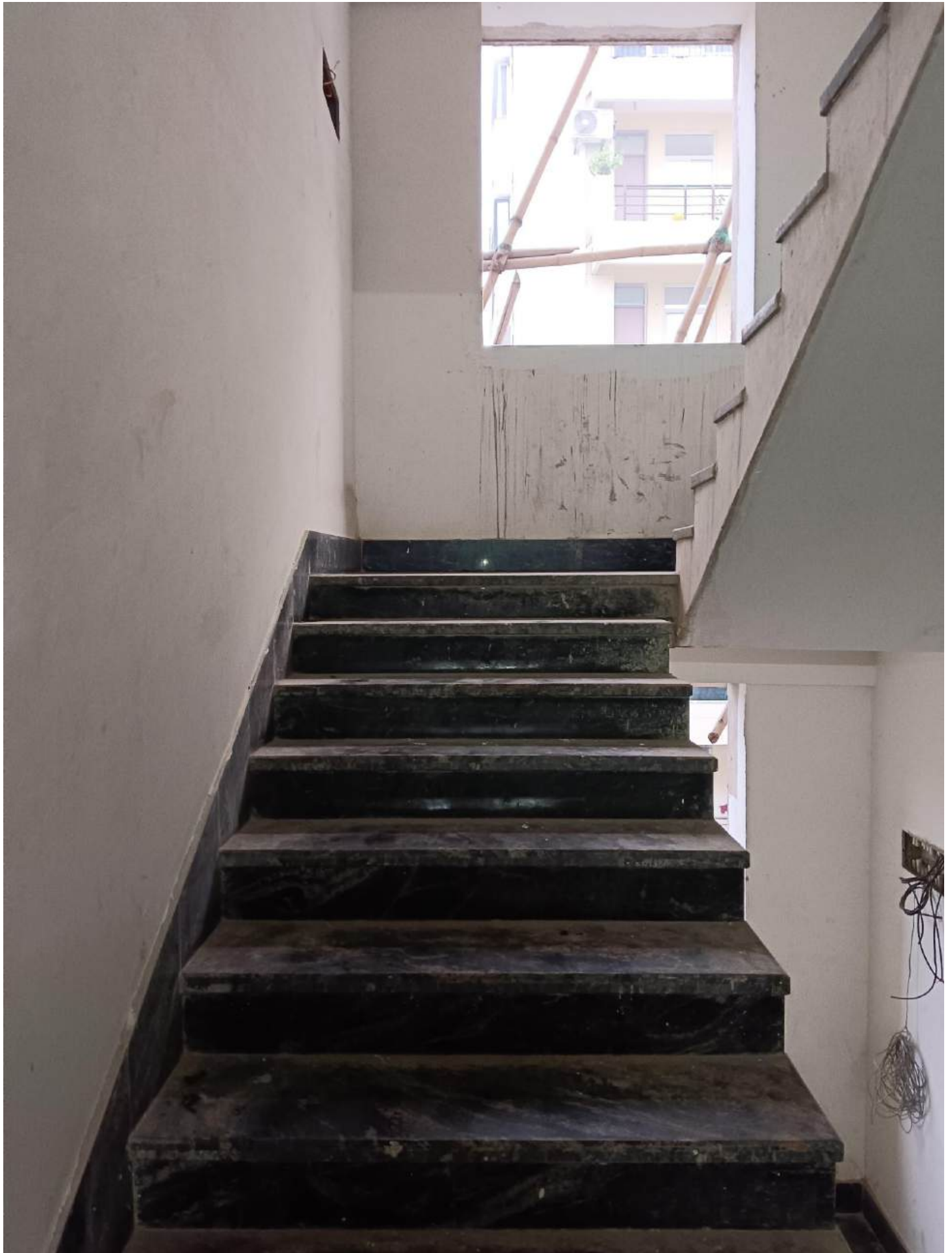
2 ND FL STAIR
