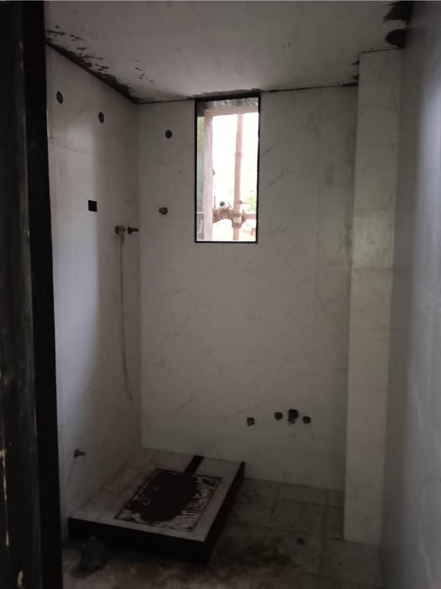
1 ST FLOOR BATHROOM
