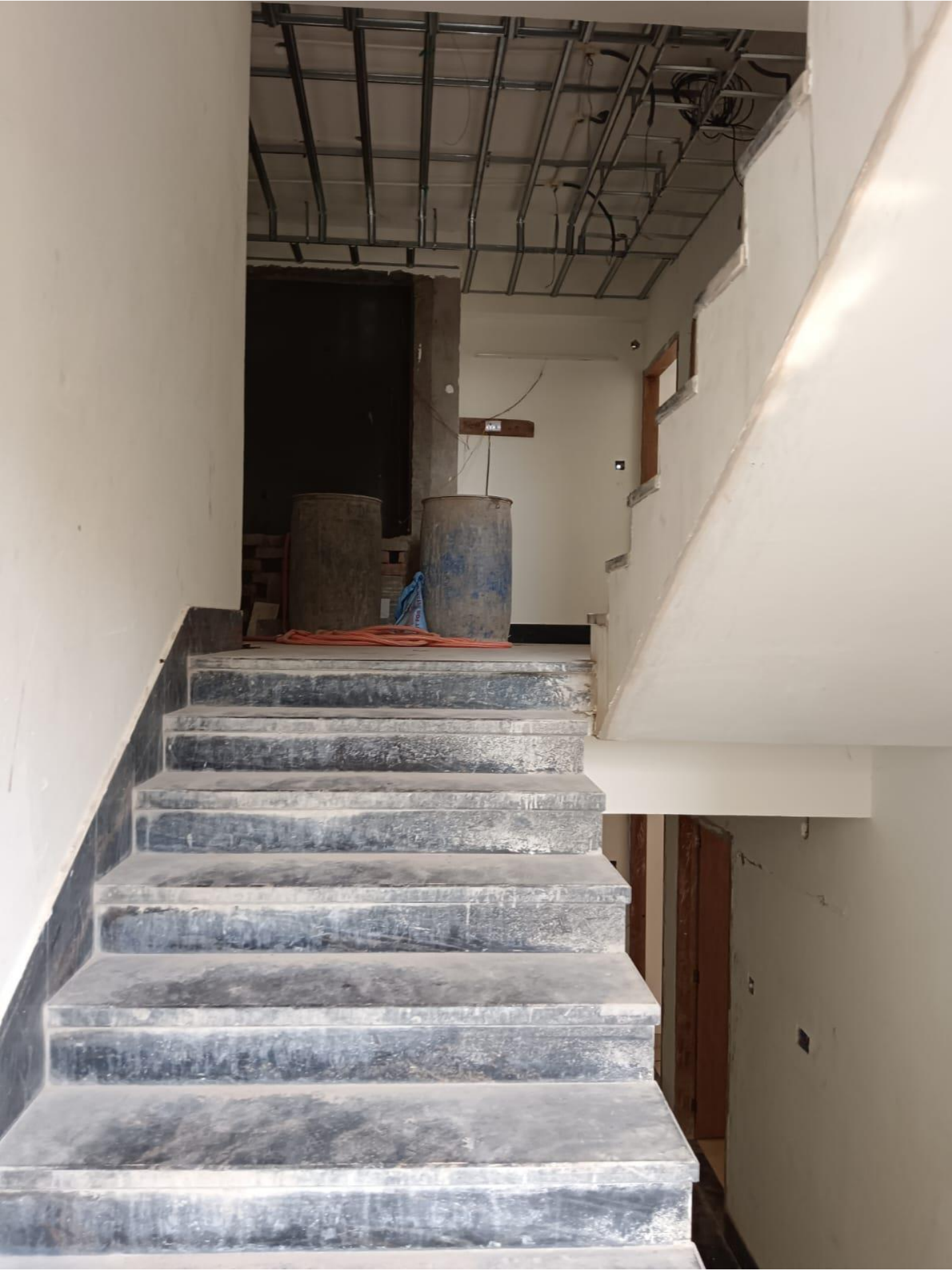
2 ND FL STAIR
