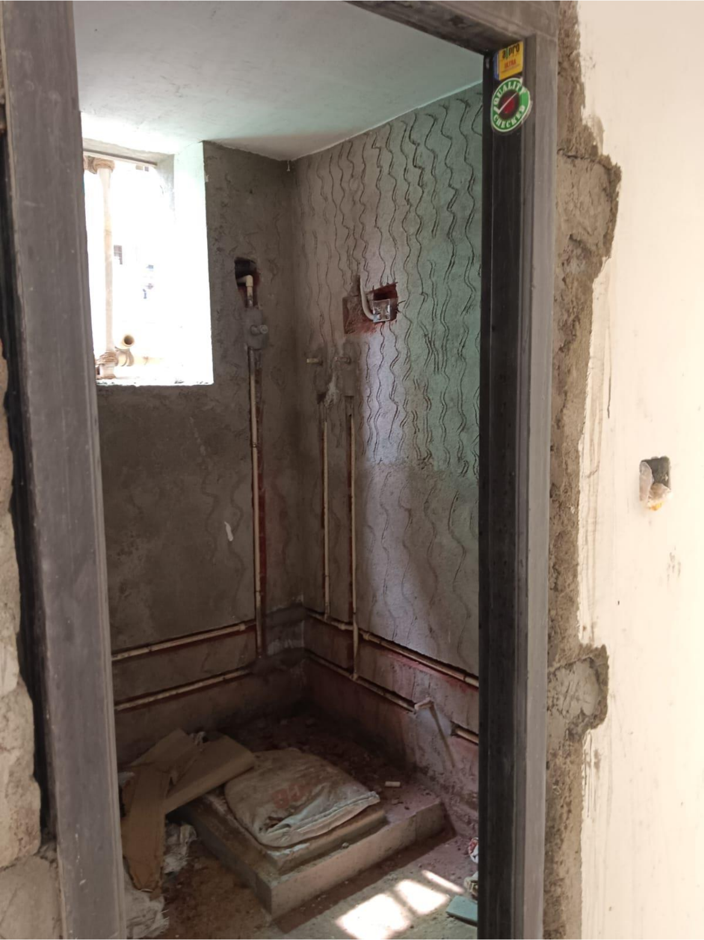
1 ST FLOOR BATHROOM
