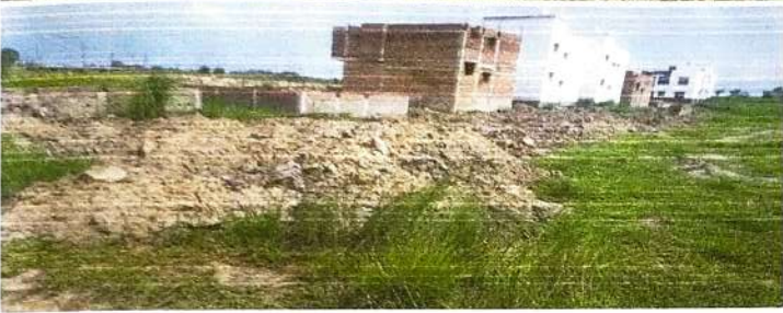
Soil Filling In Township Area
