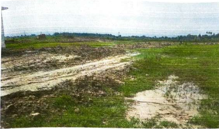
Soil Filling In Township Area
