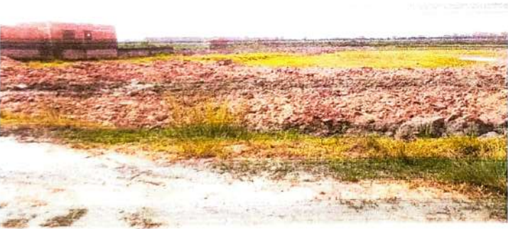
Soil Filling In Township Area
