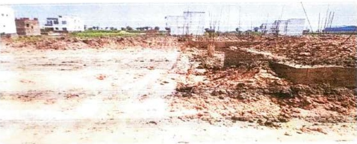
Soil Filling In Township Area
