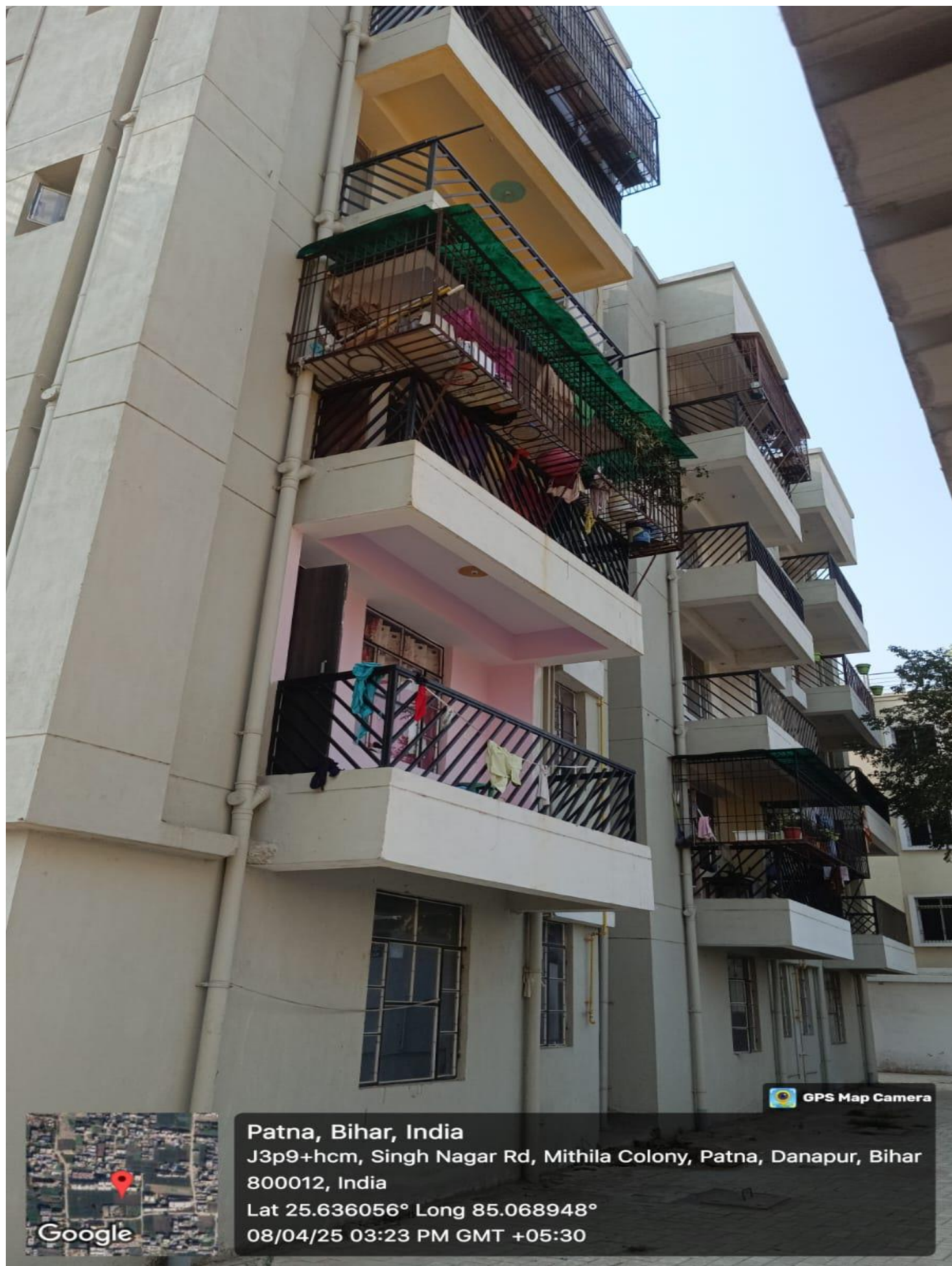
Vatika block C back side view
