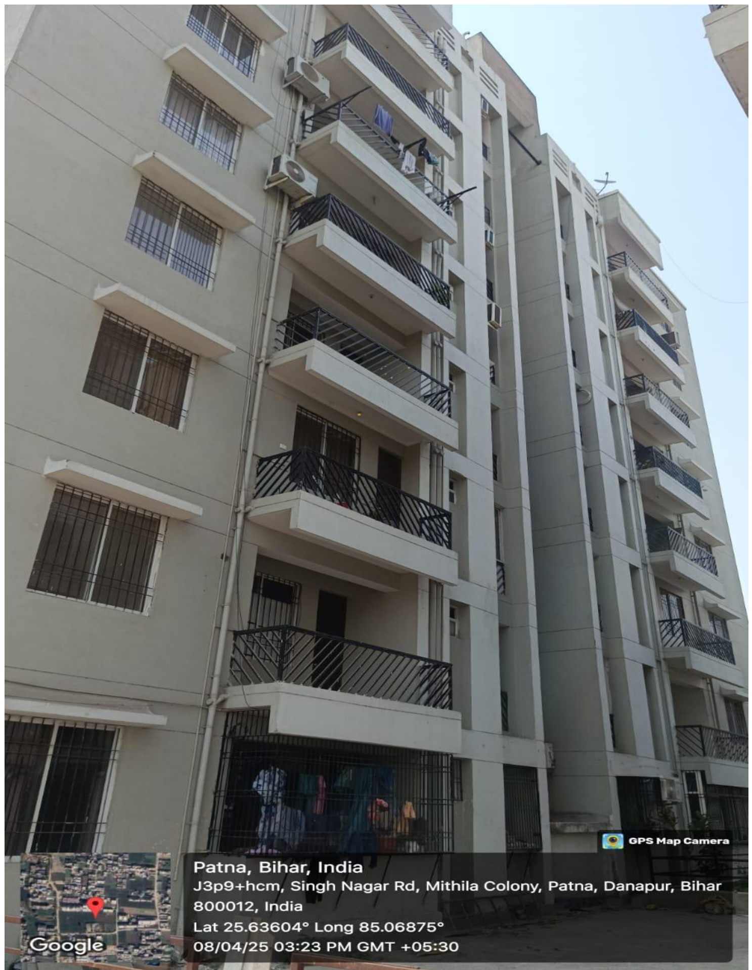
Vatika Block B backside view
