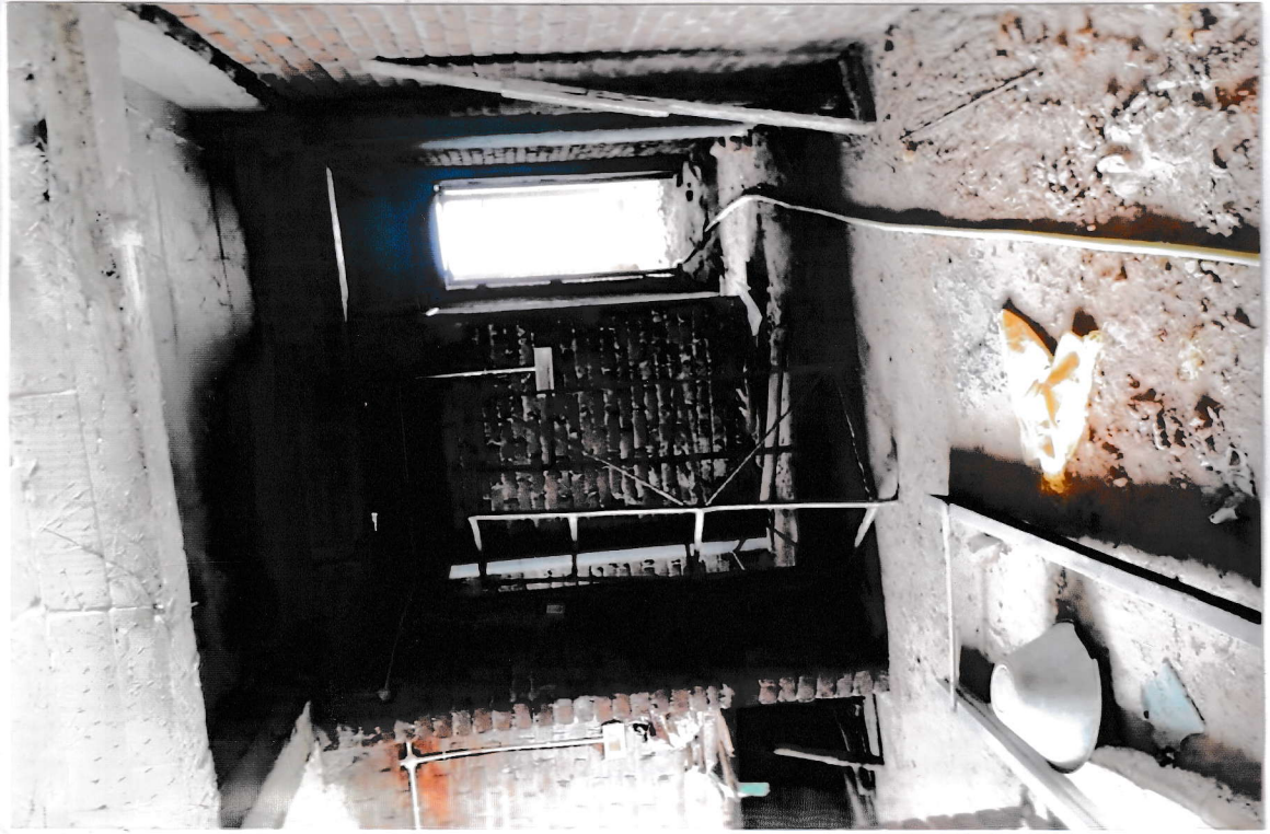
Block- A Here Is Photographs Internal Structure Work- 4 th Floor
