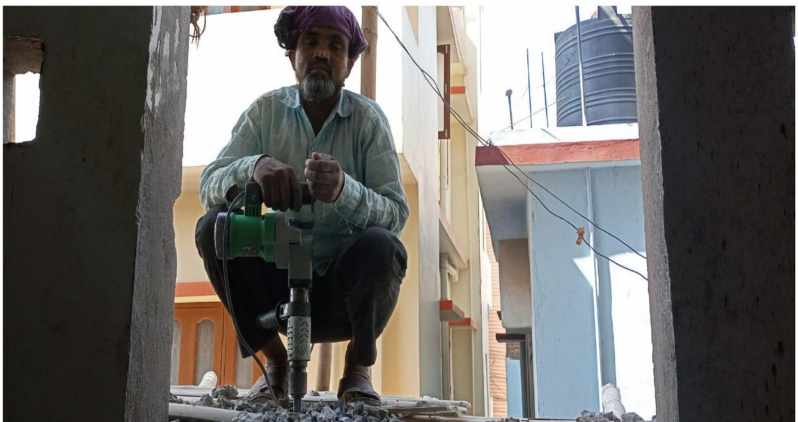
B BLOCK OUTER WALL CUTTING
