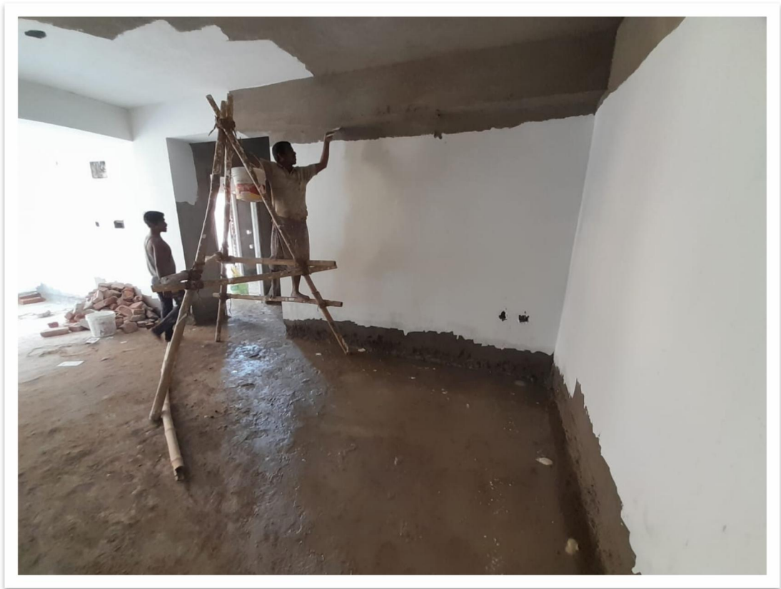
A BLOCK PUTTY WORK ON 2ND FLOOR
