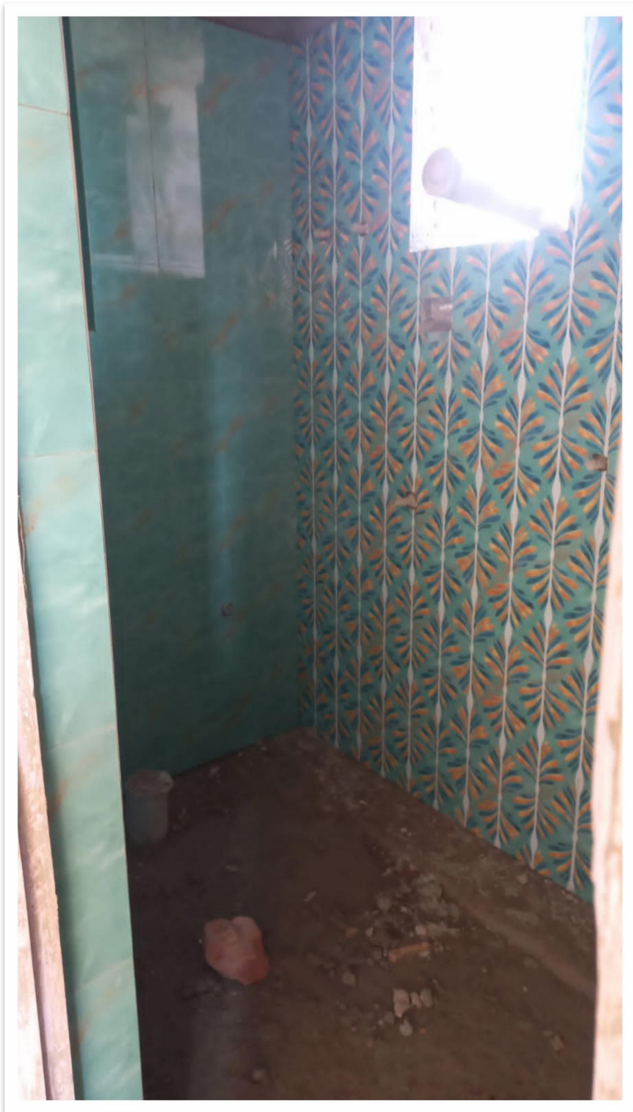
BATHROOM TILES WORK
