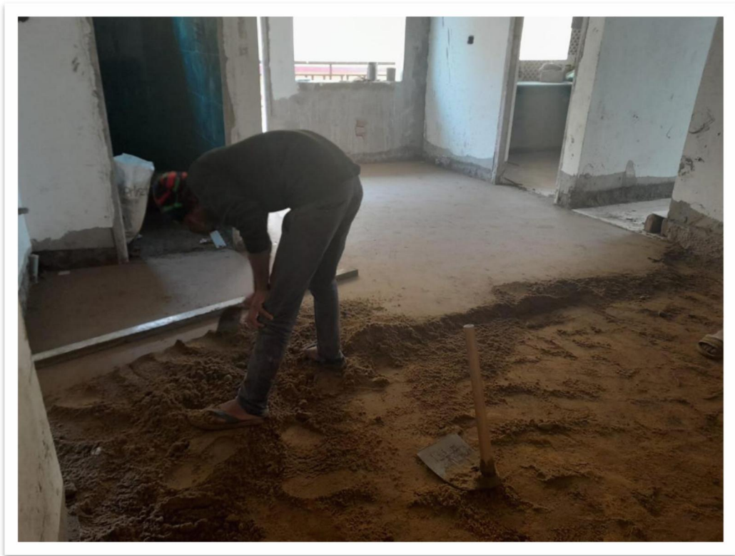
A BLOCK 4 TH FLOOR TILE WORK IN PROGRESS
