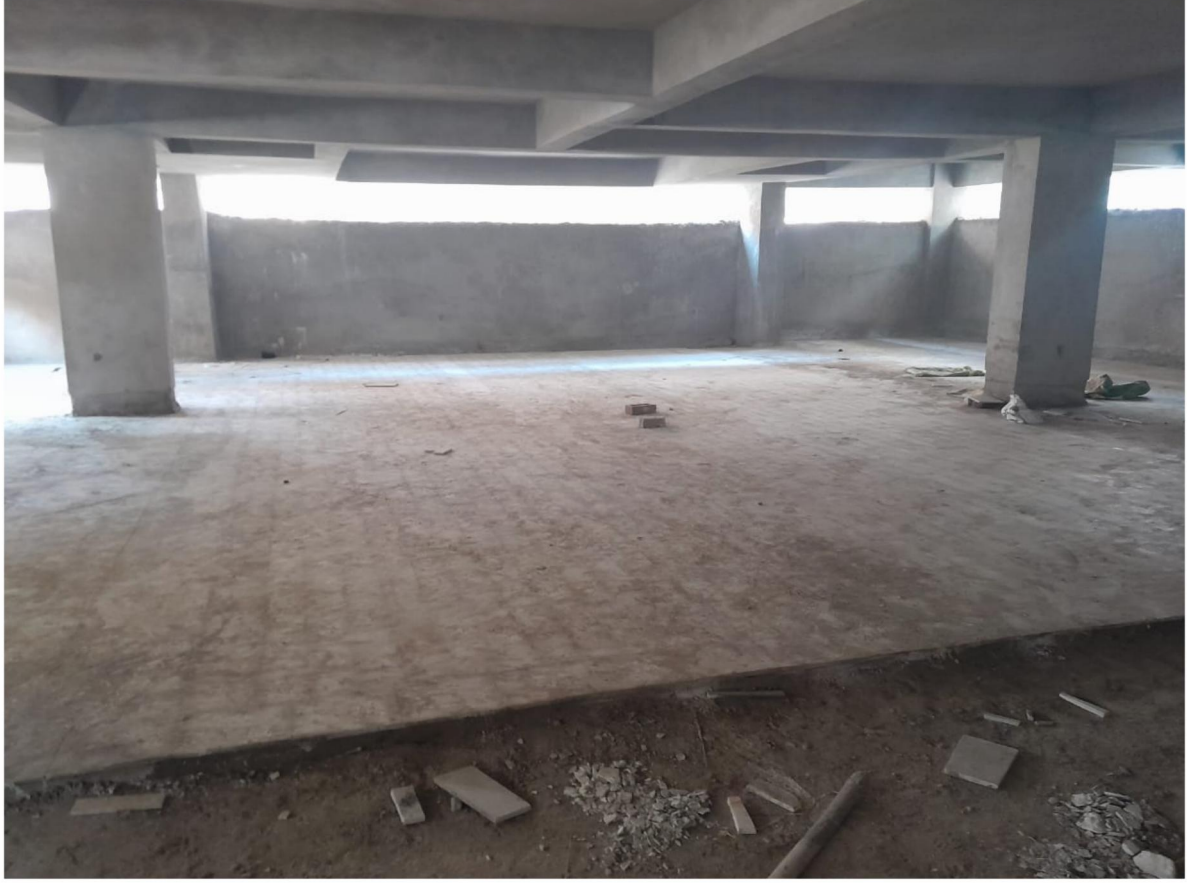
BASEMENT PARKING WORK IN PROGRESS
