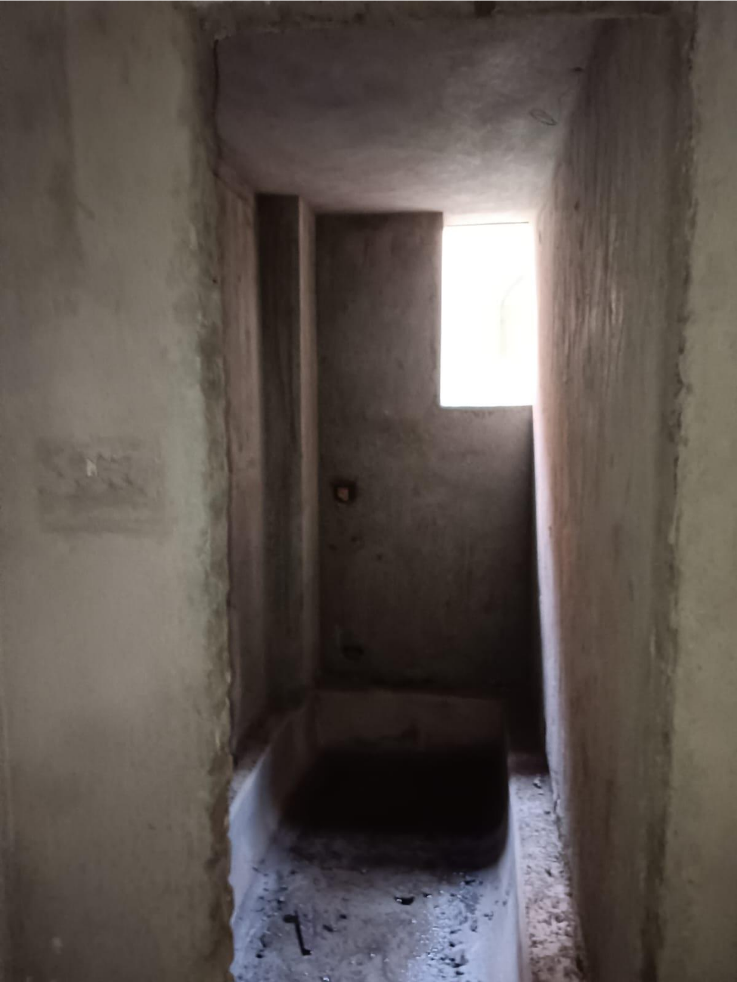
1 ST FLOOR BATHROOM
