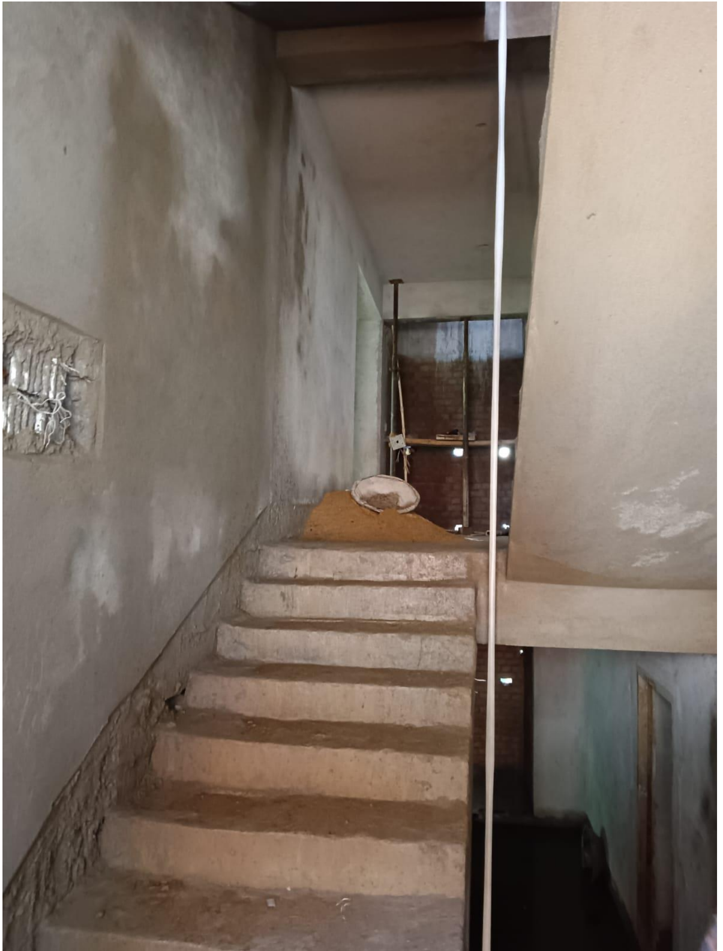
2 ND FL STAIR
