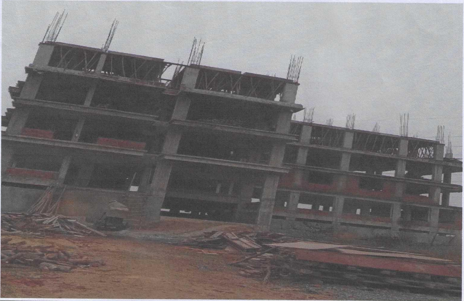
Project Site Photographs Front Elevation
