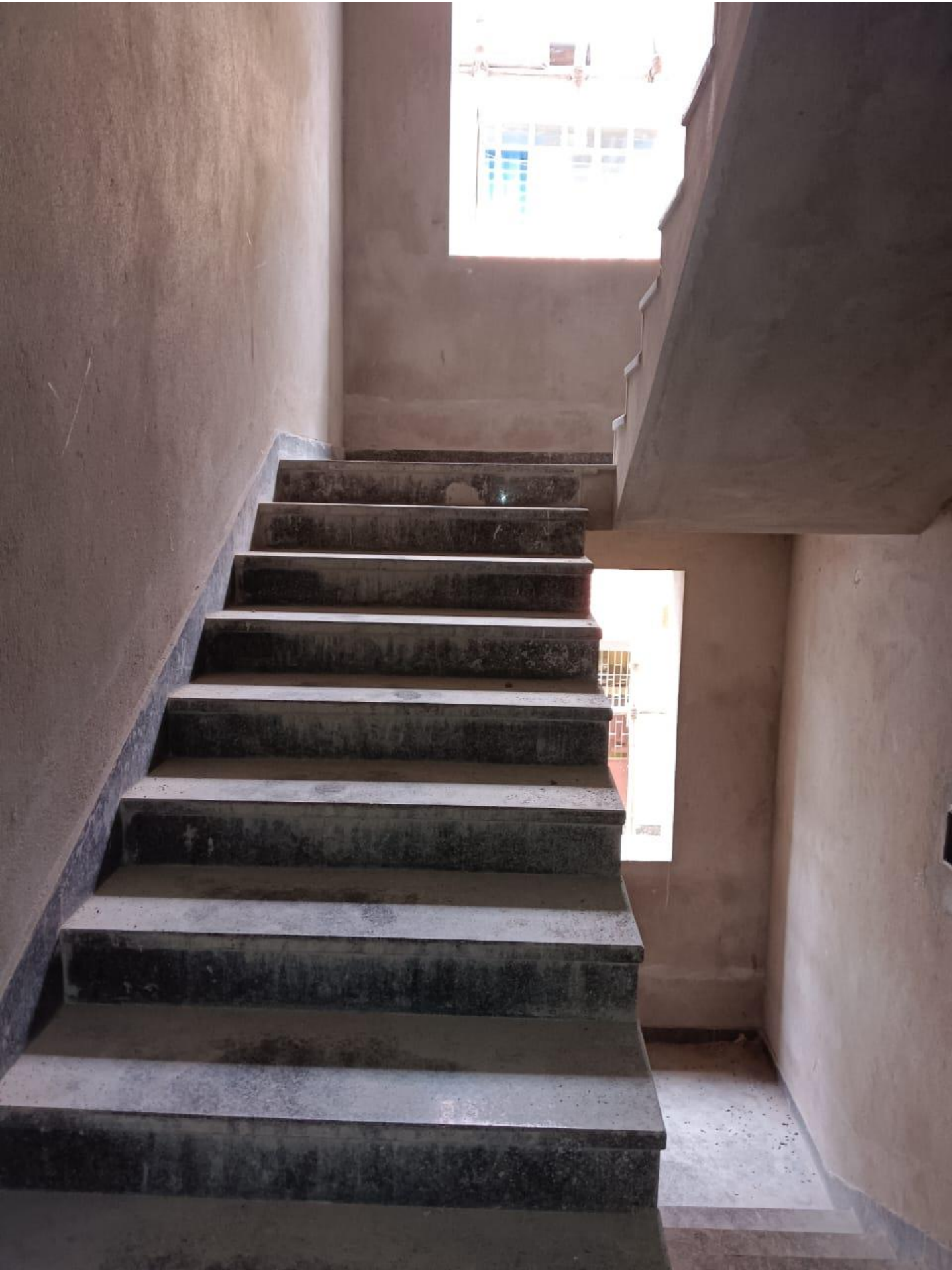
2 ND FL STAIR
