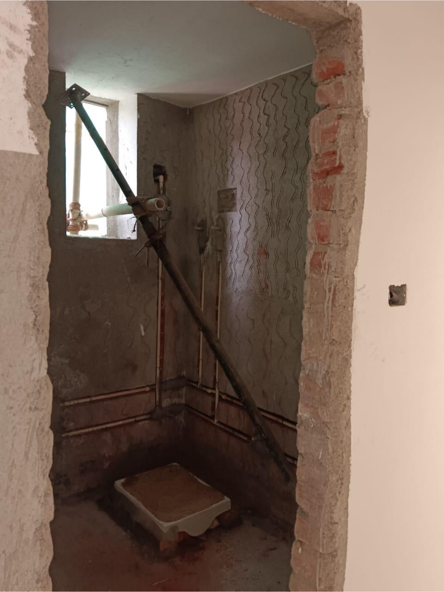
1 ST FLOOR BATHROOM
