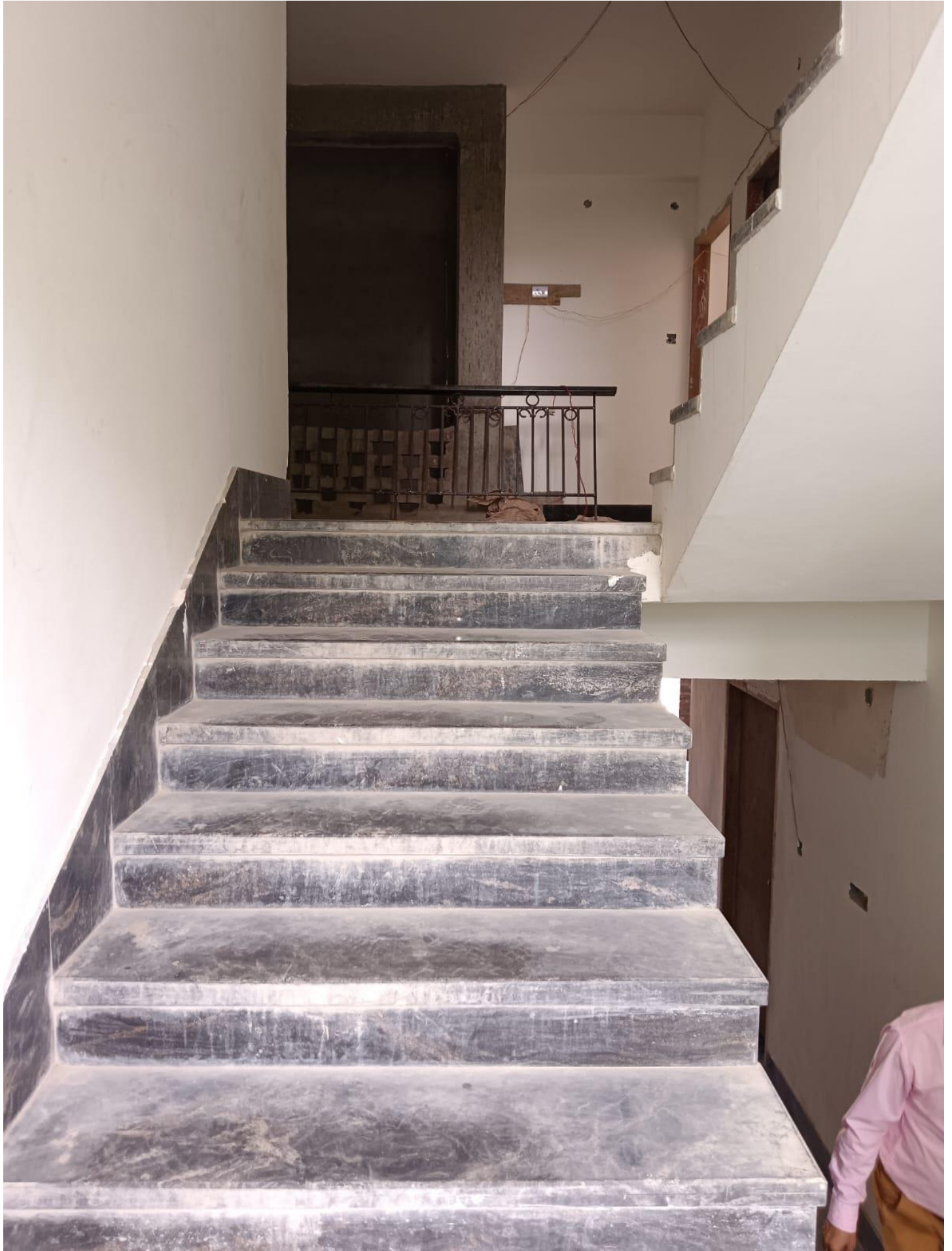
2 ND FL STAIR
